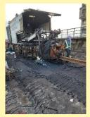
Flash butt welding was done of Head Hardened rails at the construction site of Joka Metro. The rails being used are indigenous. The results of various tests done, i.e. macro examination, transverse and hardness test were found to be satisfactory. Deployment of Flash Butt Welding machine on indigenous HH rails for Joka Metro lines will not only help in enhancing the speed but also improve the quality of work being executed by RVNL.
