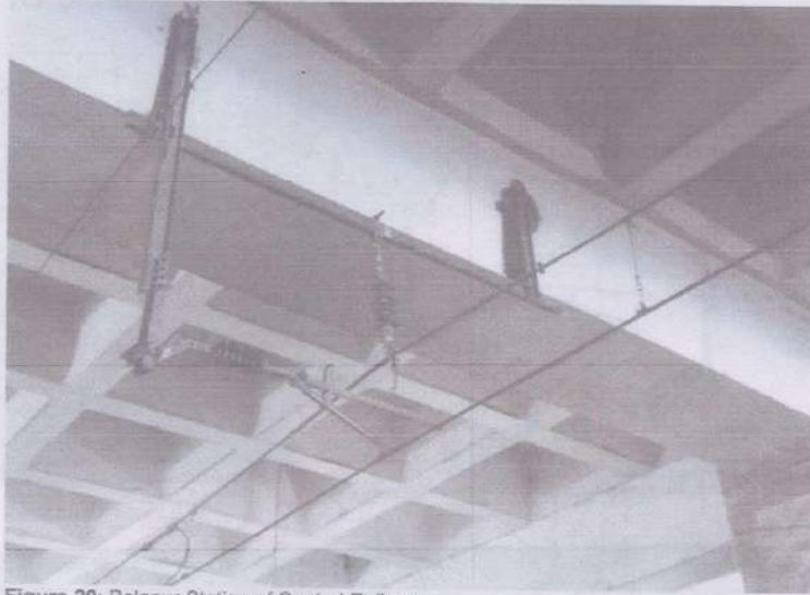
Figure 20: Belapur Station of Central Railway
