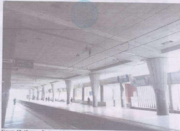
Figure 19: Kharghar Station of Central Railway
