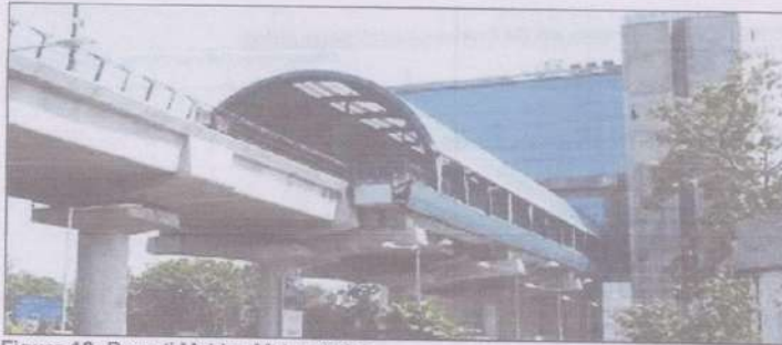
Figure 12: Pragati Maidan Metro station
